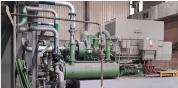
Integrally Geared Centrifugal Compressor (View-1)
