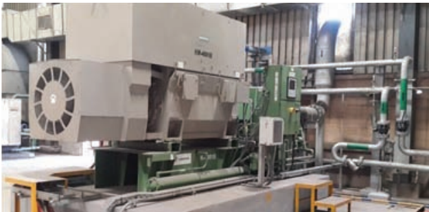
Integrally Geared Centrifugal Compressor (View-3)
